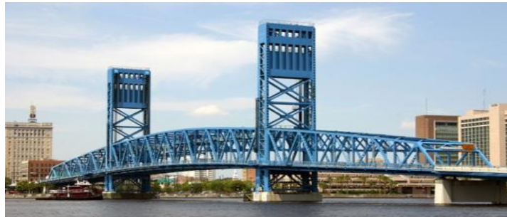
Figure 3: Main St. Bridge over the St. John’s River in Jacksonville, Florida- Built in 1941.
